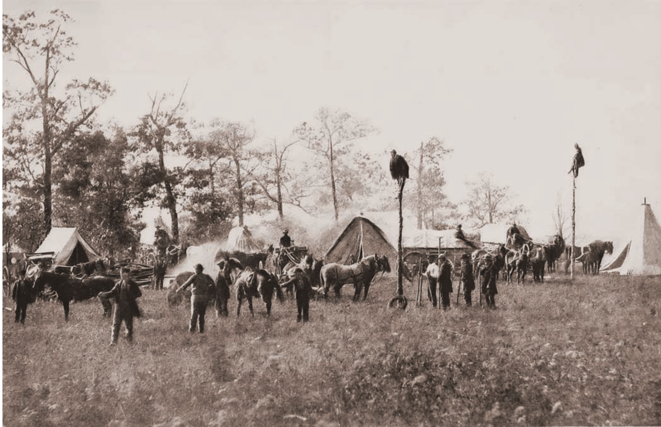
Here the camera has caught the U. S. Military Telegraph Construction Corps in action, April, 1864. The 150-odd men composing it were active throughout the war in planting poles and stringing wires in order to keep the Central Telegraph Office in direct communication with the armies at all times. Lincoln spent many an evening in the War Department Building at the capital reading the dispatches from the front handed to him by the operators. The photograph but faintly indicates the flexible insulated wire, which by this time had come into use, and in the picture is being strung along by the two men on the poles and the three in advance of them in the left foreground.
